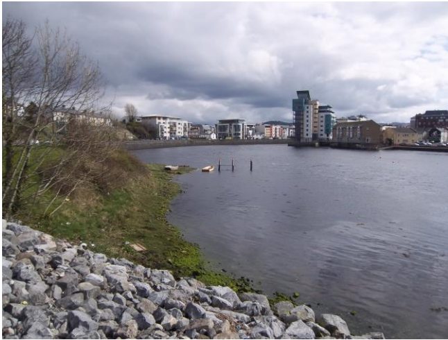
Image 6.1 : Garavogue River upstream of Hughes Bridge, showing artificial south bank and earth north bank
