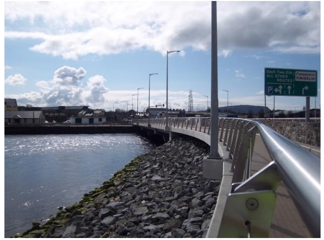
Image 6.2 : Rip rap present on Garavogue River upstream of Hughes Bridge
