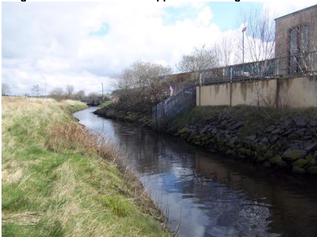
Image 6.5 : Copper River bank reinforcement on the south bank and earth banks on the north bank
